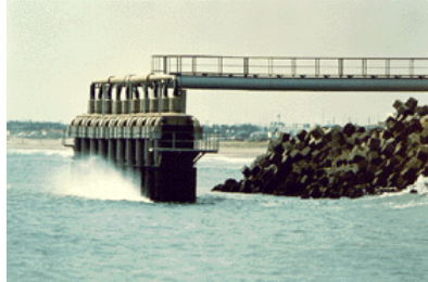
Fig.3 Wave-breaker type wave power generation system with constant-pressure-tank
